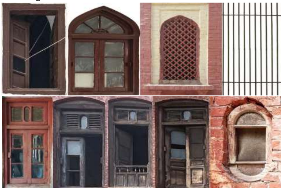
Figure 9. Exterior Façade Windows
